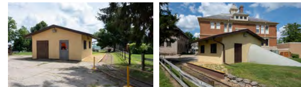
Existing Depot Building Mine Entrance and Train Depot Area
