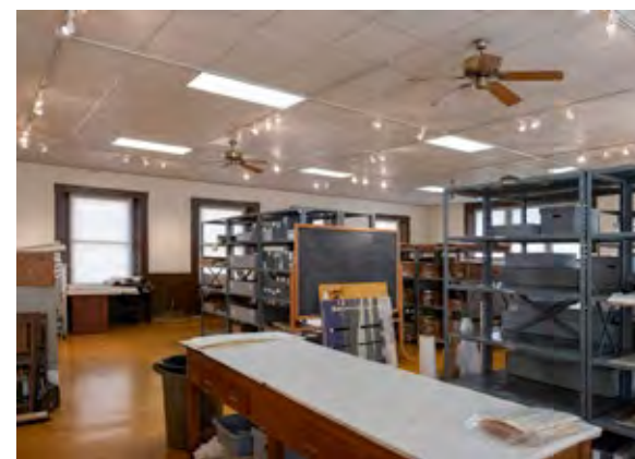
Upper Level Lacks ADA accessibility Maintain existing function as employee-only space for Museum Archive
