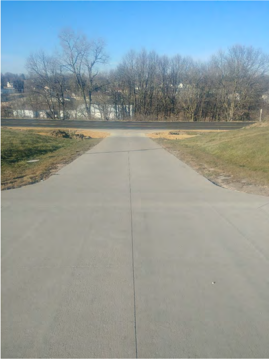
Driveway viewing north toward Bus 151
