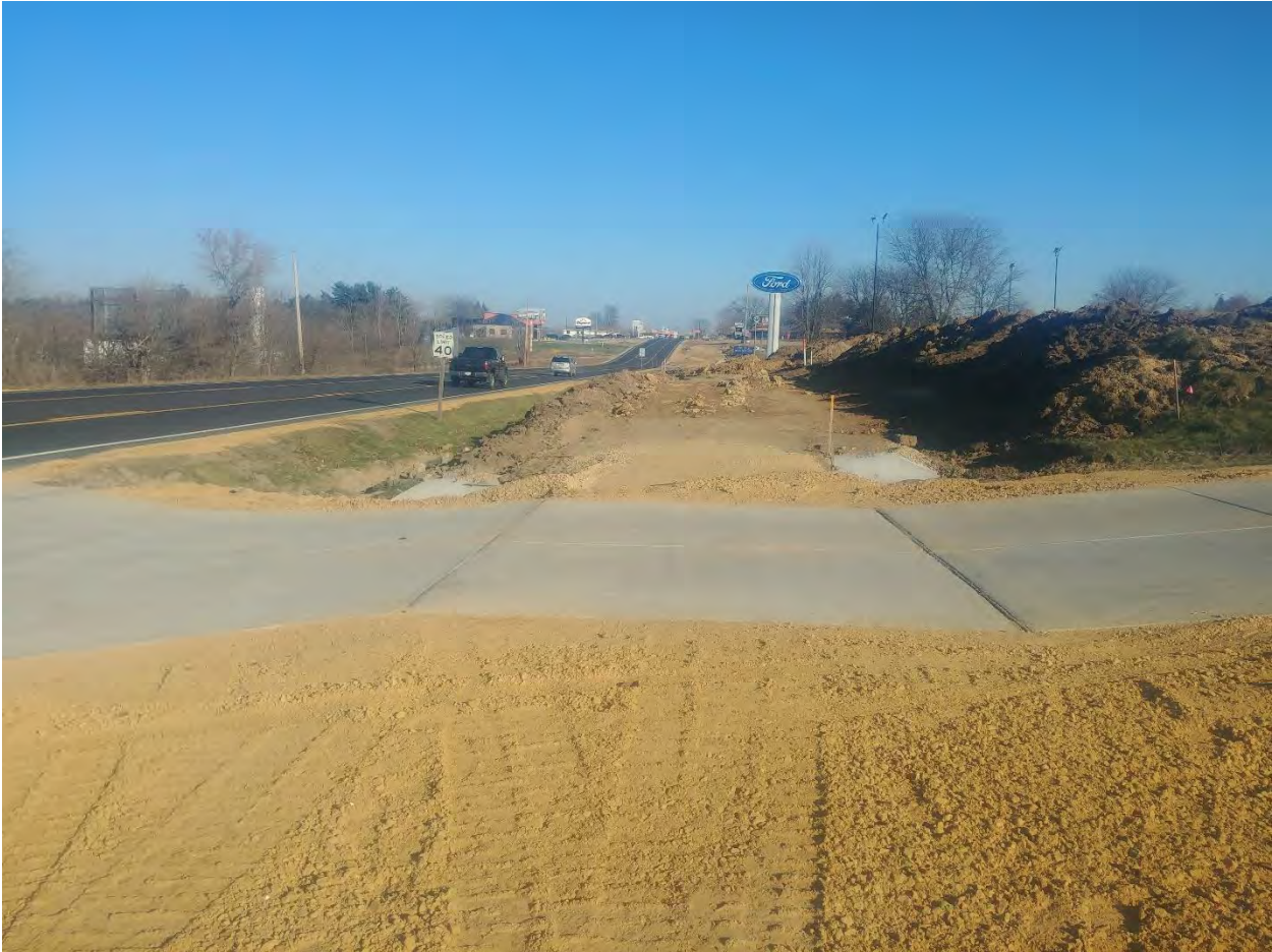
Trail crossing driveway viewing east
