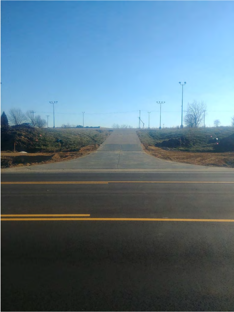
Driveway viewing south from Bus 151
