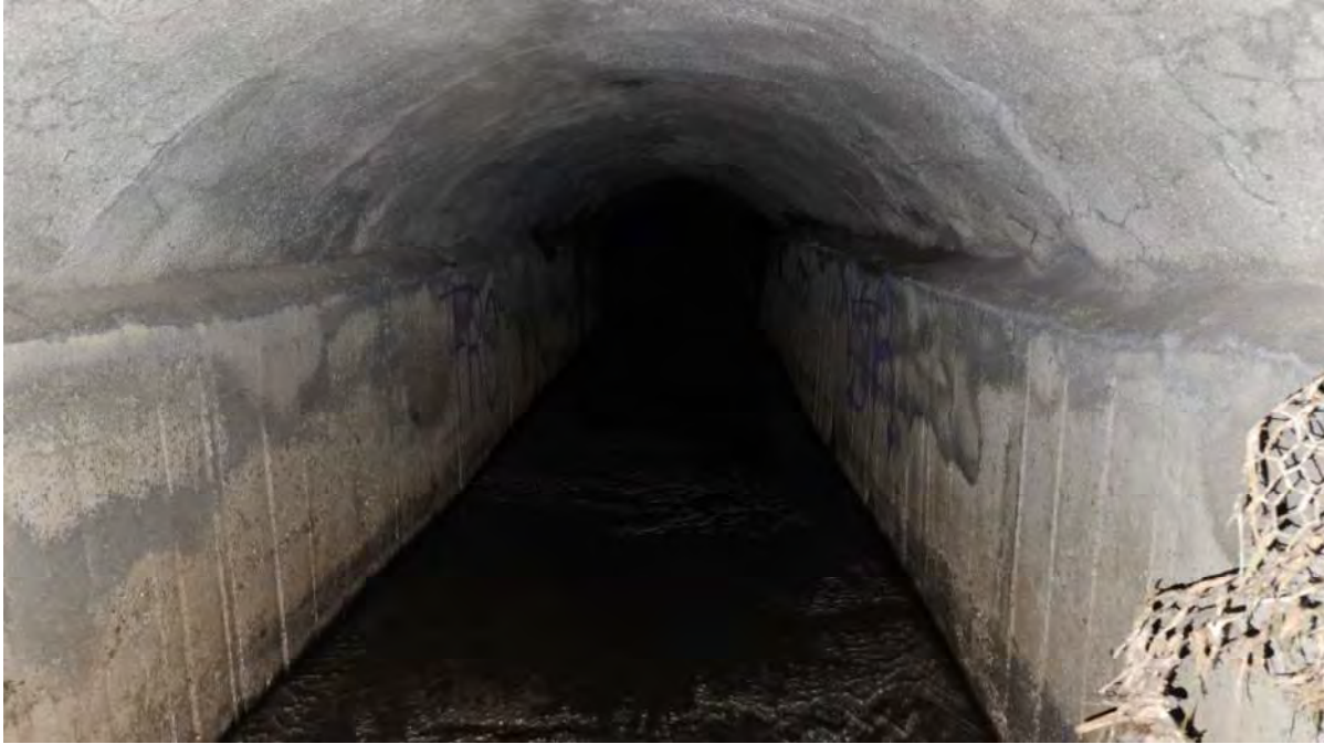
Photo looking down outlet culvert
