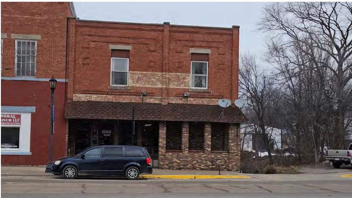
Photo of the south exterior elevation showing a widening gap between the subject building and adjacent building to the west.
