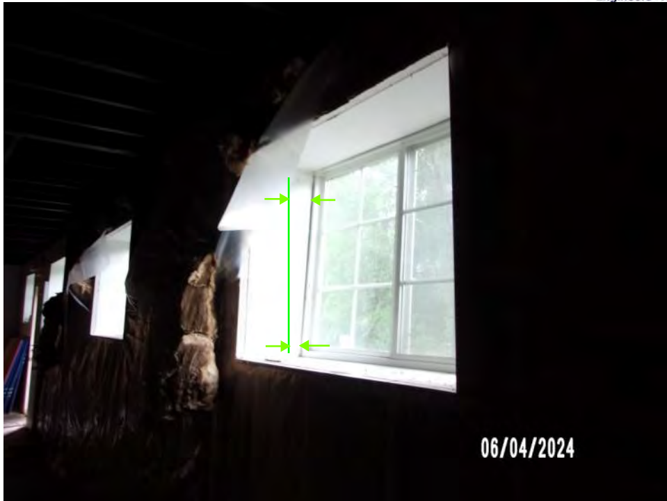
Photo 15 – Windows set in wood wall lean to the east
