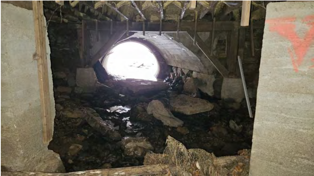
Photo of the entry culvert
