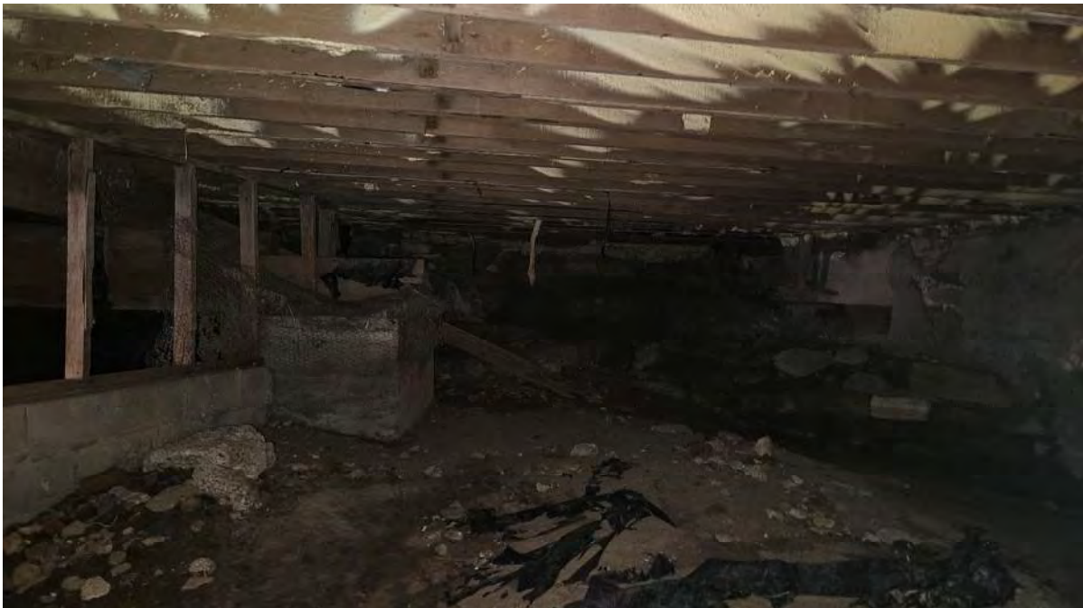
Photo looking south at the southwest corner of the foundation
