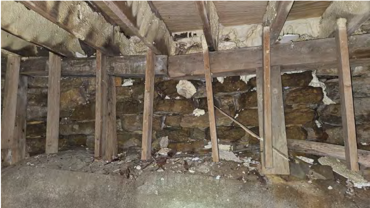
Photo showing timber floor support system
