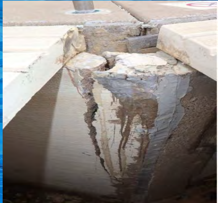
South wall transition corner
