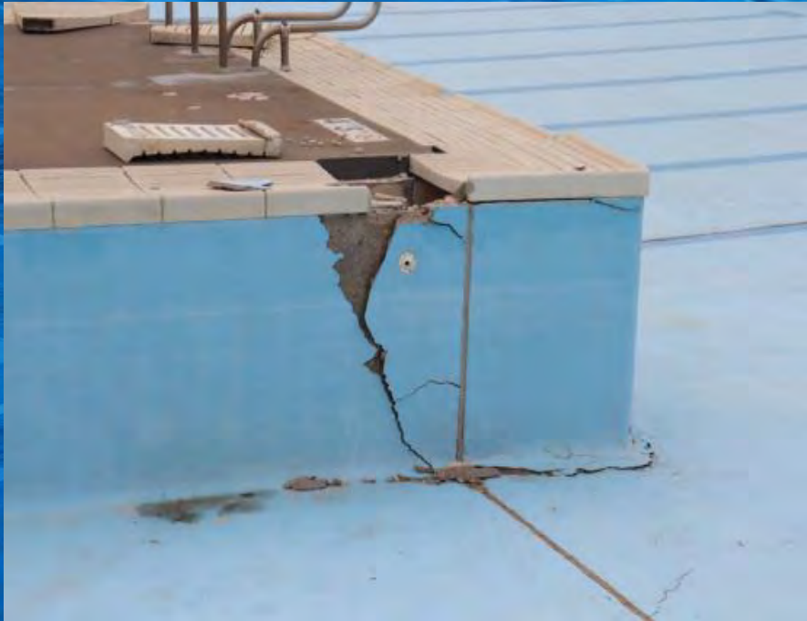
East slide area wall
