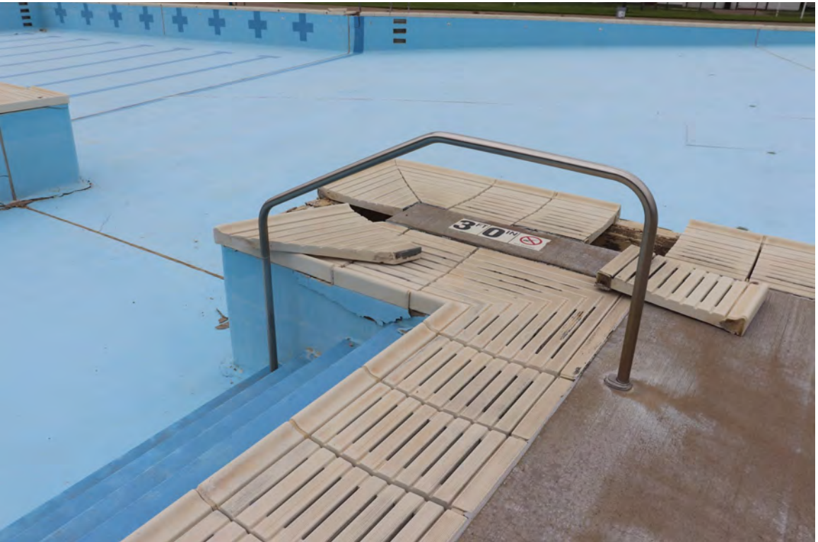
Figure 15 Alternate view illustrating slide area exit stairs and proximity
