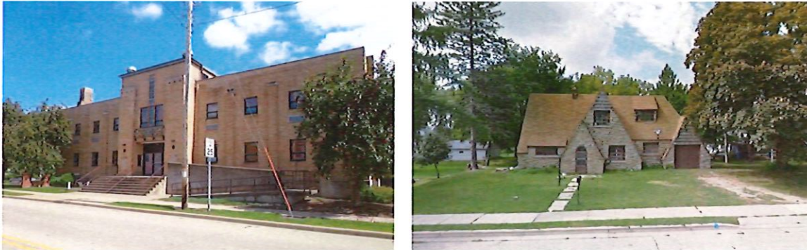
Platteville Civic Center/National Guard Armory at 475 N. Water Street (left); Paul Steuhl House at 1050 N. 2nd Street (right).
